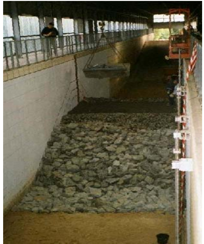
Fig. 1. Construction of the rubble mound breakwater in the wave flume.
