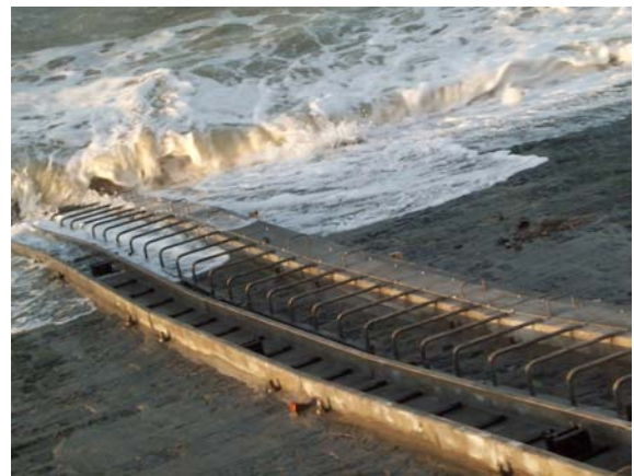
Fig. 1. Installation ducts at the measurement site in Oostende.
